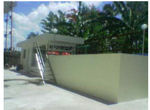
Pharmaceutical Laboratory SBR Process Capacity: 48 m 3 /day
